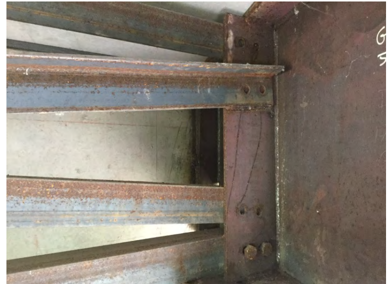
Downstream left bank girder bracing welded
