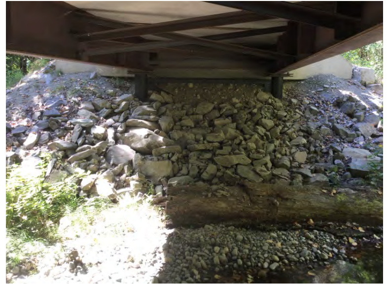
Right Bank Abutment when facing downstream
