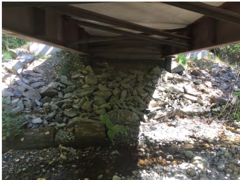
Left Bank Abutment when facing downstream
