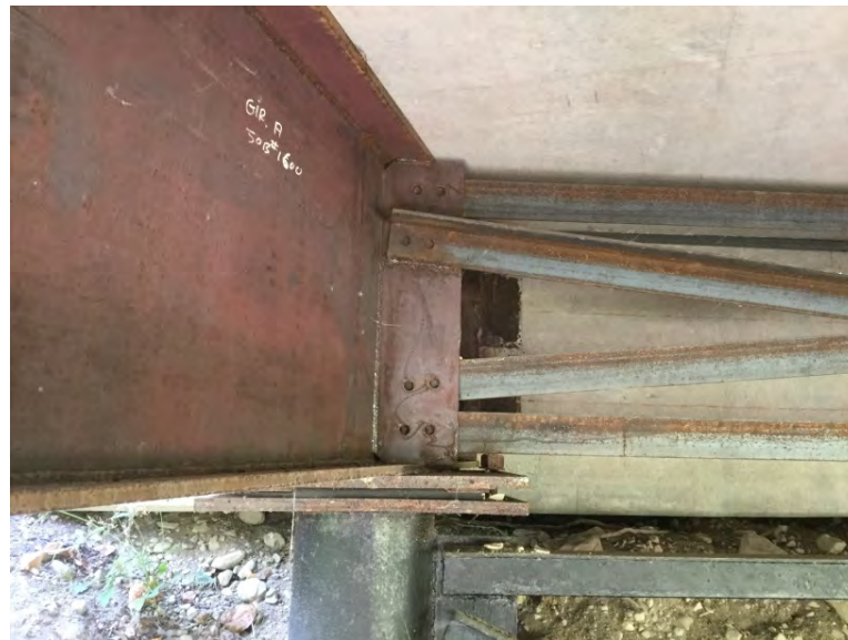
Downstream right bank girder bracing welded
